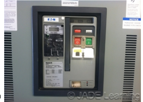
Branch-circuit disconnects rated 1000 amps or more and installed on solidly grounded wye electrical systems of more than 150 volts to ground require GFPE.
