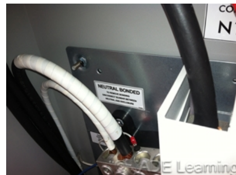
Generators now must be marked to indicate whether or not the generator neutral is bonded to the generator frame.
